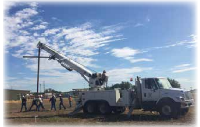
CVE crews help erect four, 26 foot tall metal crosses located when you enter Artesia from Roswell and Carlsbad on Highway 285, and from Loco Hills and Hope on Highway 82.
